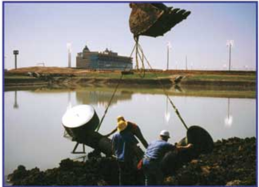
Construction Phase of Lone Star Park in Grand Prairie
